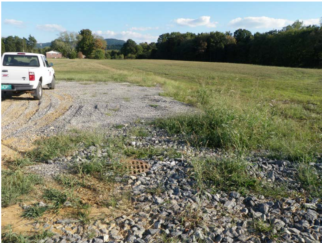
Photo 4. Upgradient (southeast) view of WWC-1/UDF-1 at Sta. 13+75L showing catch basin this feature drains into.
